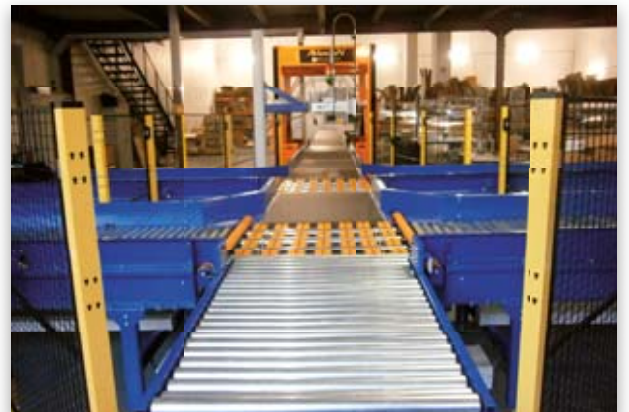
Installation with 4 outlet lines
