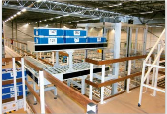
Feed conveyor on mezzanine
